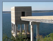
Williamson County Regional Raw Water Line Stillhouse Hollow Lake Intake Structure
